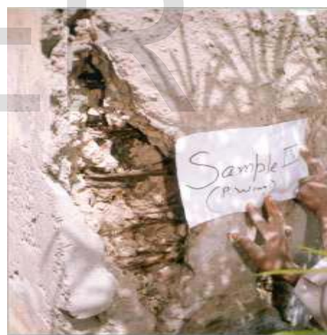
Photo-2 Cracks in Column of school building due to corrosion of reinforcement
