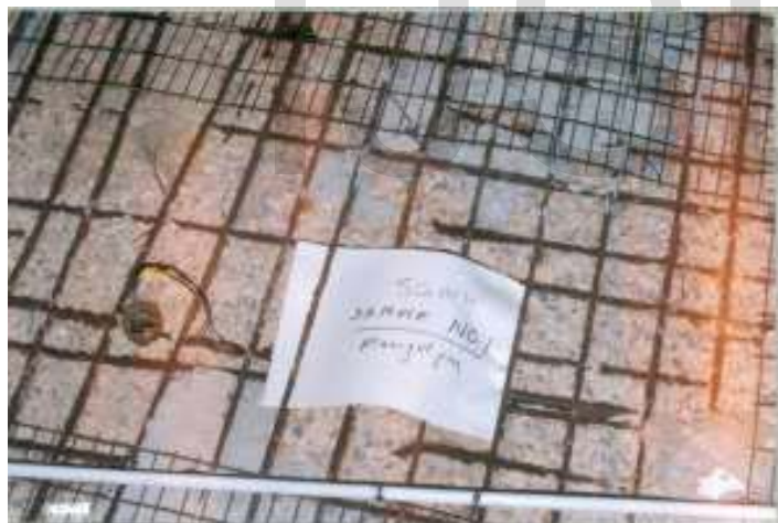
Photo-1 : Ceiling of a hospital building where plaster has got delaminated from reinforcement due to corrosion of reinforcement
